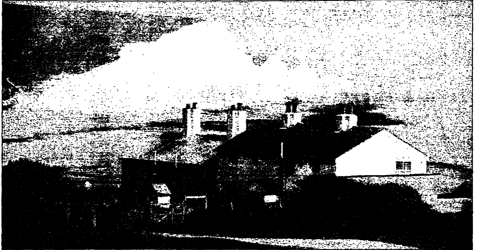
The cottages above Cuckmere Haven that have been saved from the sea, despite lobbying from conservationists to let nature run its course
